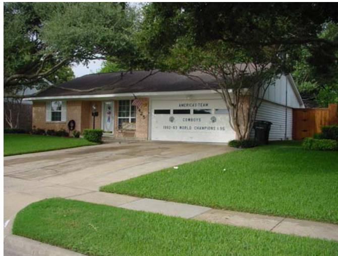
Figure 8 – Rehabilitated home in Meadows Addition
