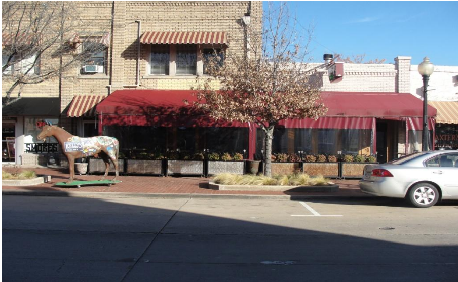
Existing front facade of 1422 K Avenue
