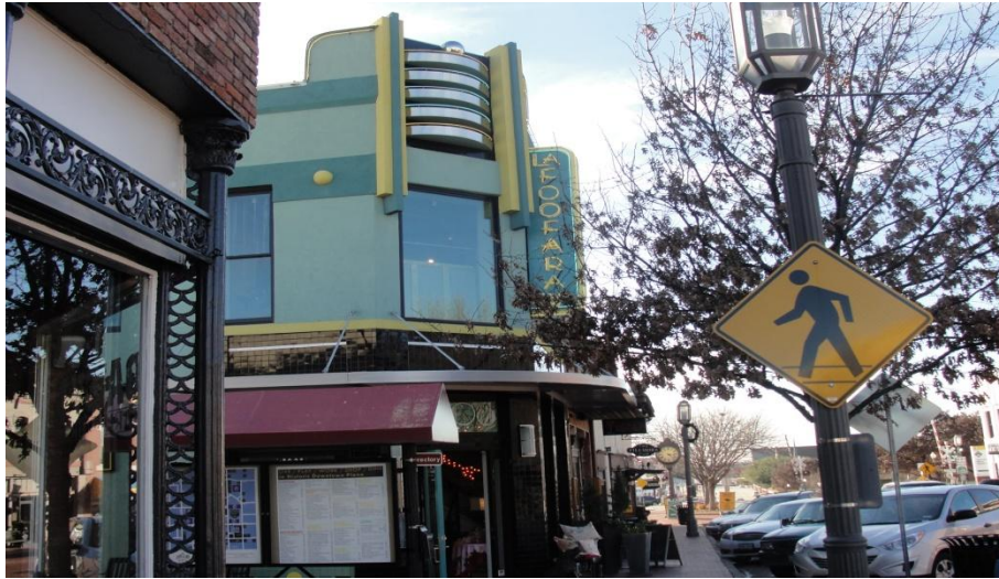
Existing front and side facades of 1008 E. 15th Street
